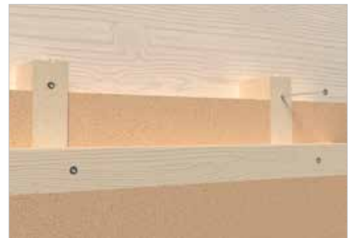
TTUFS screws in light wall framing.
